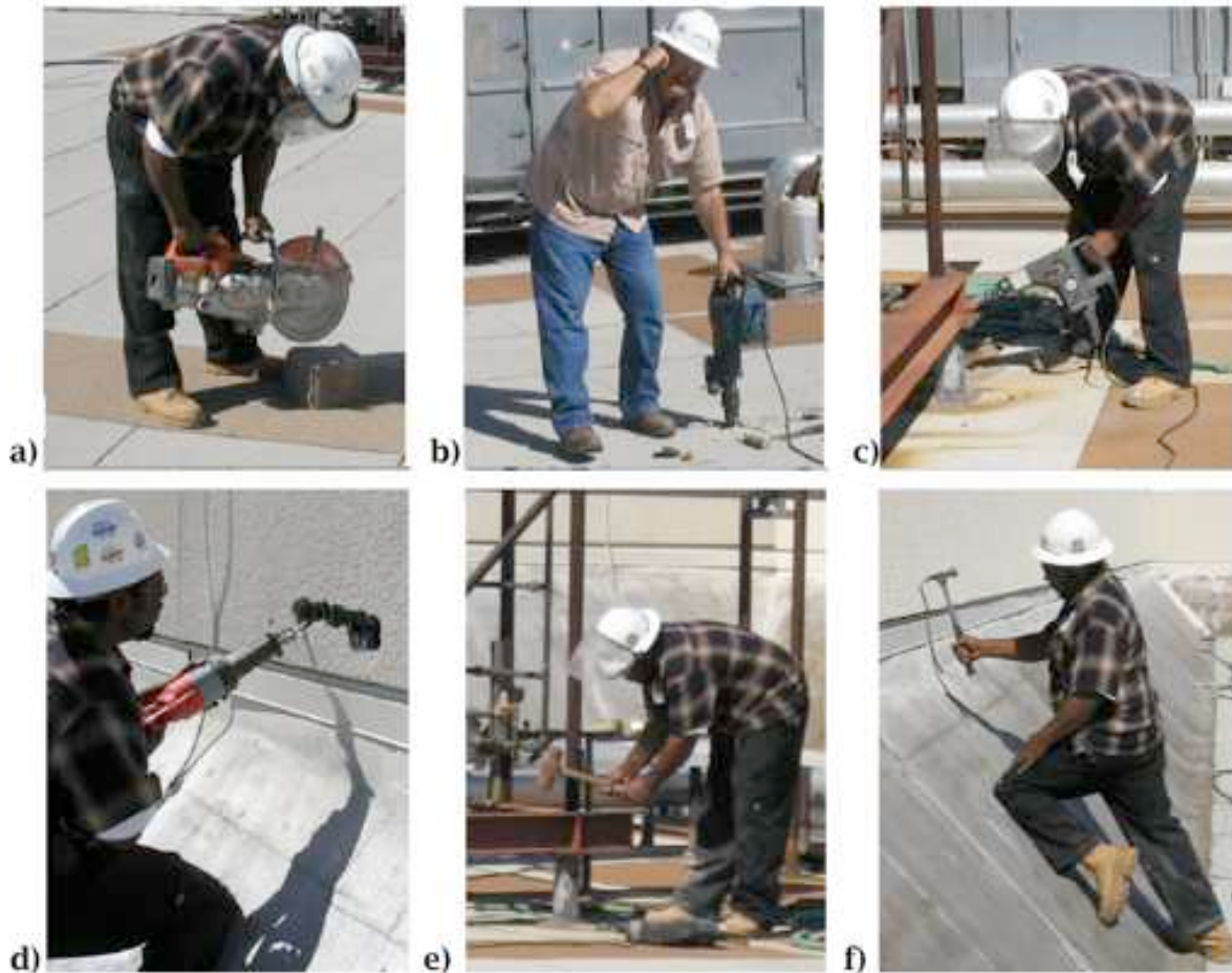
Figure 6: Tool Simulations: (a) concrete saw, (b) chipping (rotary) hammer, (c) slag hammer, (d) sawsall (reciprocating saw) and manual tools; (e) sledge hammer and (f) claw hammer. (g - fastening device not pictured)
