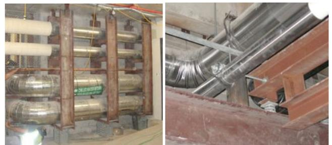
Fig. 6. Vibration Isolated Pipe Racks.
