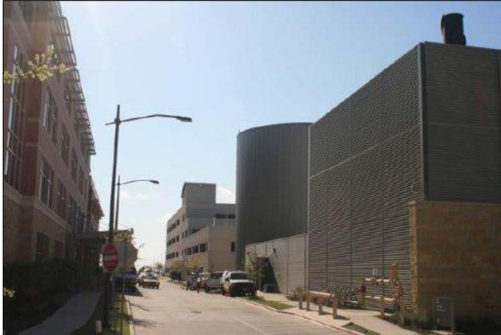
Figure 1. Power plant (right) and medical office building (left).
