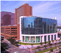
Texas Heart Institute - Denton A Cooley Building, Houston, TX
