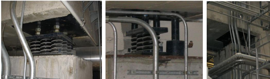
Figures 7, 8 & 9 – Spring Isolators, Viscous Damper (center) and Conduit Flanking Isolators
