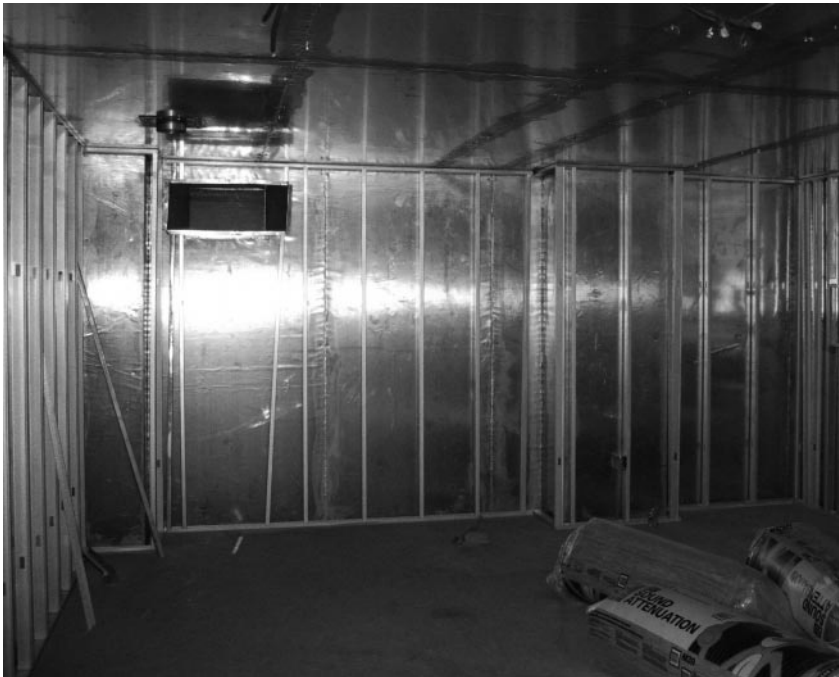
Figure 9. Partition framing and shielding
