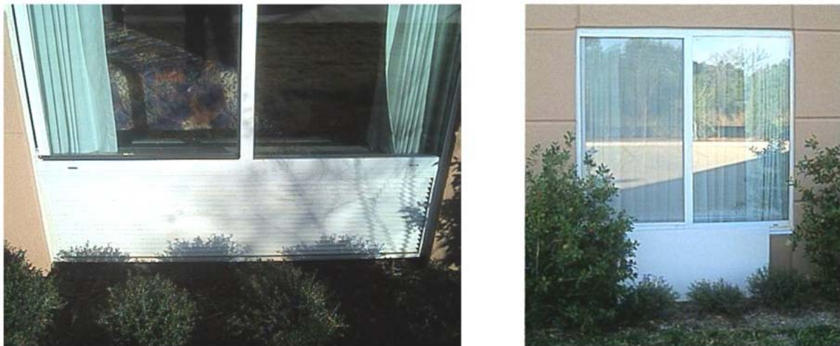
Figure 3: outside views of air conditioners without baffle (left) and with baffle (right)
