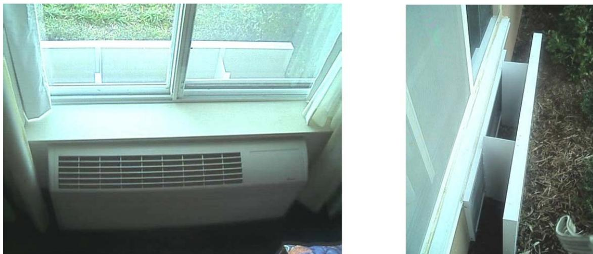
Figure 6: inside (left) and outside (right) views of typical air conditioner with baffle
