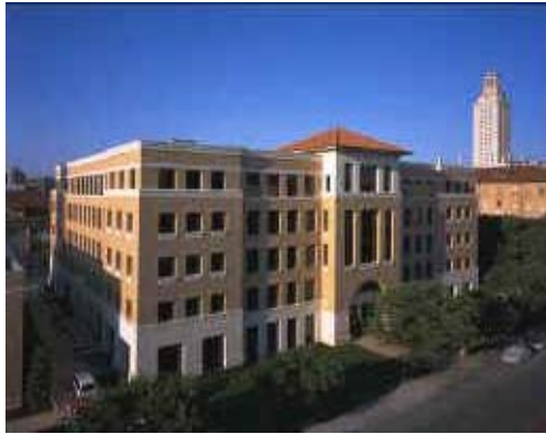
Figure 1A. ACES Building, North View
